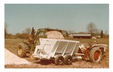
In 1976 C. U. invented the wet lime spreader allowing farmers to backhaul truckloads of inexpensive lime and stockpile it in corners of their fields for use when conditions allowed. Subsequent improvements achieved accurate fertilizer spreading with rates as low as 125 pounds per acre
